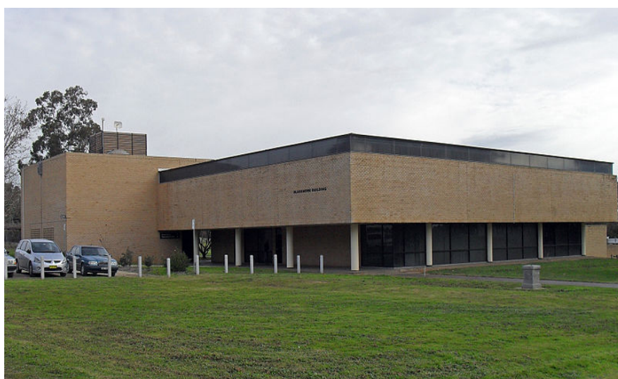
Blakemore Building , Charles Sturt University, South Campus.
